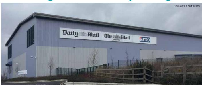
were able to start from scratch. The only water we use in the production process is rainwater and the building is heated during the day by the heat given off by the presses at night. This means free heating in the building, without the need for gas."
